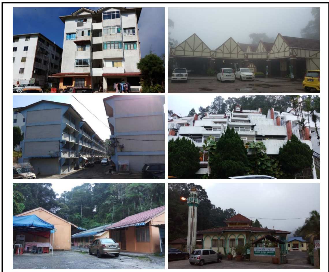
Figure 11: Modern buildings in Fraser's Hill (Author, 2018).
